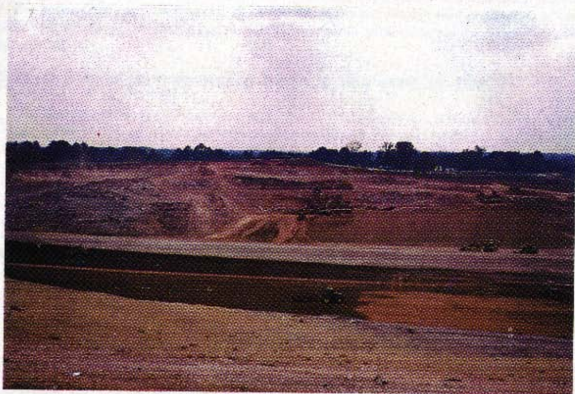
SANITARY LANDFILL SITE UNDER PREPARATION
